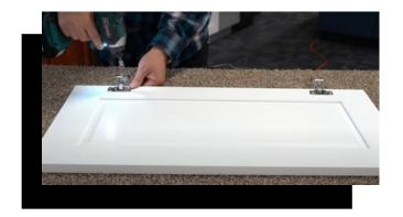
8. Place the hinge into the pre-drilled hinge holes and screw in place. Make sure that you are using the round-headed, short screws and not the flat-headed screws so that the screw won't run through the door. Repeat the same steps for installing the other remaining hinges
