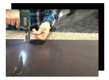
6. Place the back panel piece down, fitting into the pre-cut channels of the side panels, making sure that the panels are all flush and sitting flat before securing the side panels to the back panel with brad nails.
