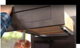
14. Once both slides have been secured to the drawer box, pull out both slides and place on the drawer box, make sure to fit the drawer box's back notches to the slides first. Pull the slides all the way up to the drawer clips until you hear a "click" sound confirming that the slides are secured to the clips.
