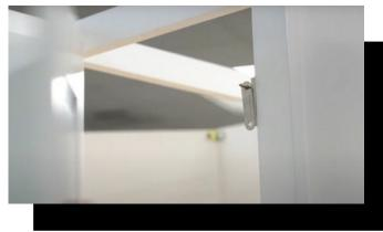
10. Next, stick the thin metal piece with a screw through one of the holes onto the magnetic white piece on the frame. Press the door lightly into the screw to create an indent on the door to map out where to screw in the metal bit. Before screwing on, double check that the screw length isn't too long, so that it won't run through the door.
