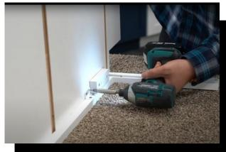
3. Further secure the side panel to the frame using the provided metal L brackets, placing one at the top and one at the bottom of the frame. Repeat steps 2 - 3 for the other frame and front side panel piece. Making sure to that the grooves of the two pieces line up to each other before securing in place.
